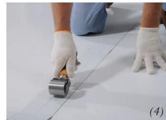
Peel & Seal PowerBond® White 250 installs in just four easy steps. (1) Wipe surface clean with acetone. (2) Peel back release liner. (3) Apply to seam of panels. (4) Roll seam for a tight and secure seal.
